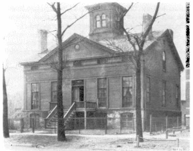
In 1935, the Historic American Buildings Survey, a project of the federal government, recorded the house in photographs and measured drawings. Much of the detailing was gone, including the front portico which had been removed when the house was moved in 1872.
